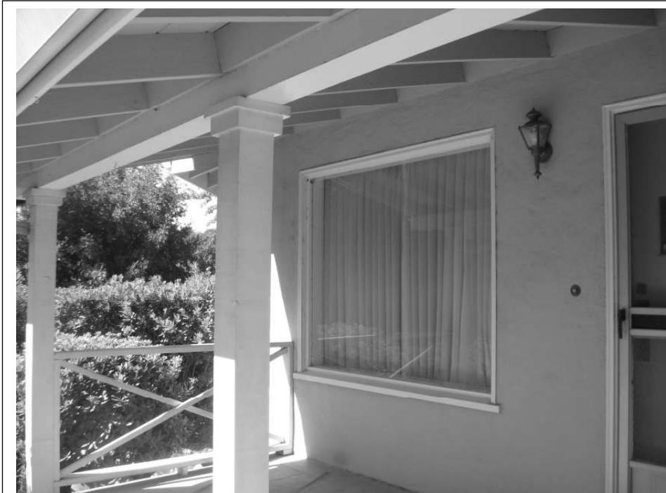
Photo 5: View of the porch showing exposed rafters.
