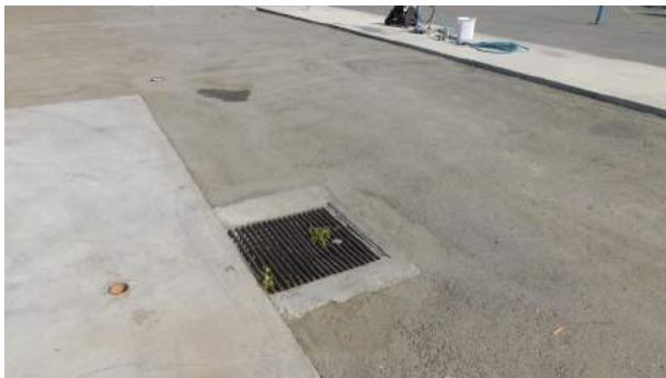
Storm water drain between propane tank and RV check-in area
