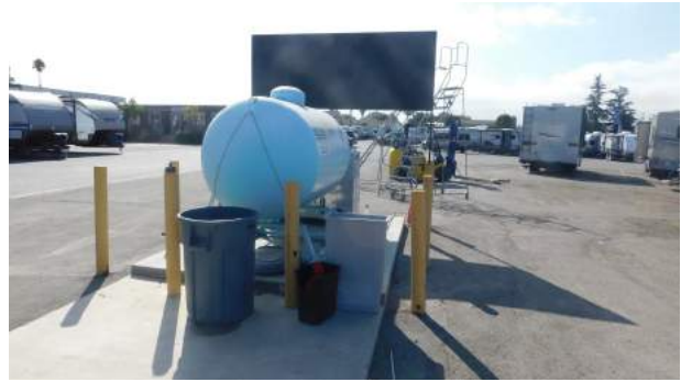
Above ground propane tank
