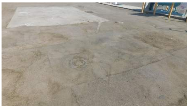
Random concrete slab with evidence of an abandoned underground hydraulic lift
