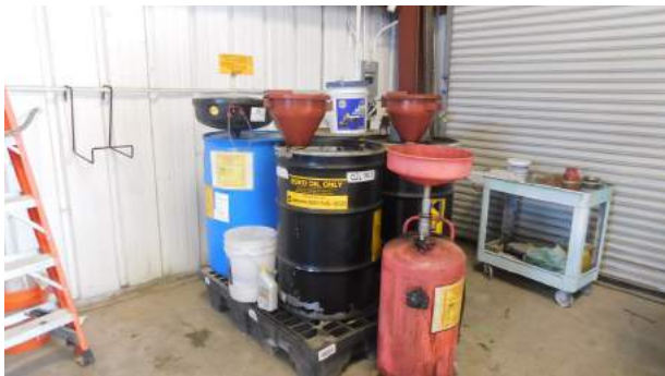
55 gallon and 30 gallon drums of used oil on secondary containment - service center
