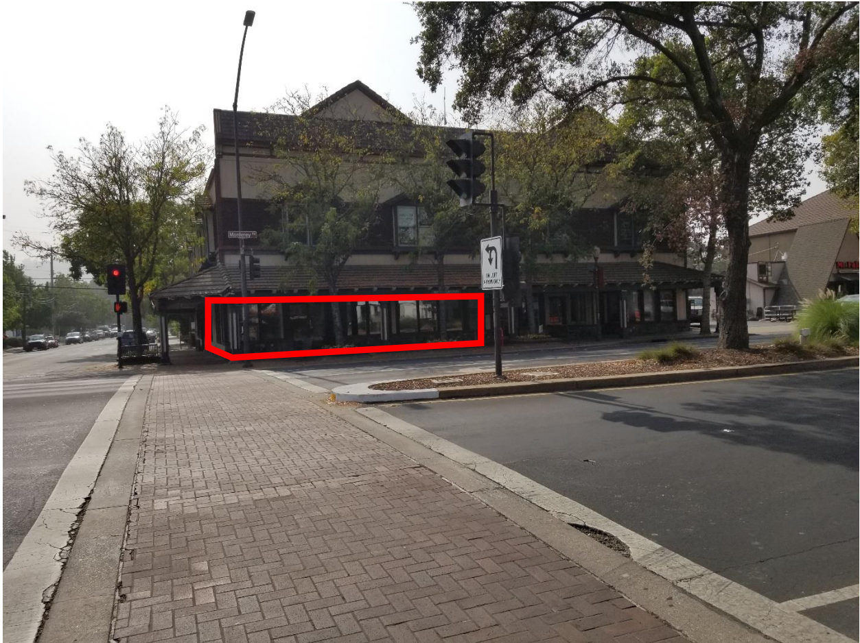
View from across Monterey Road Looking West (East facing side of 17415 Monterey Road Building)
